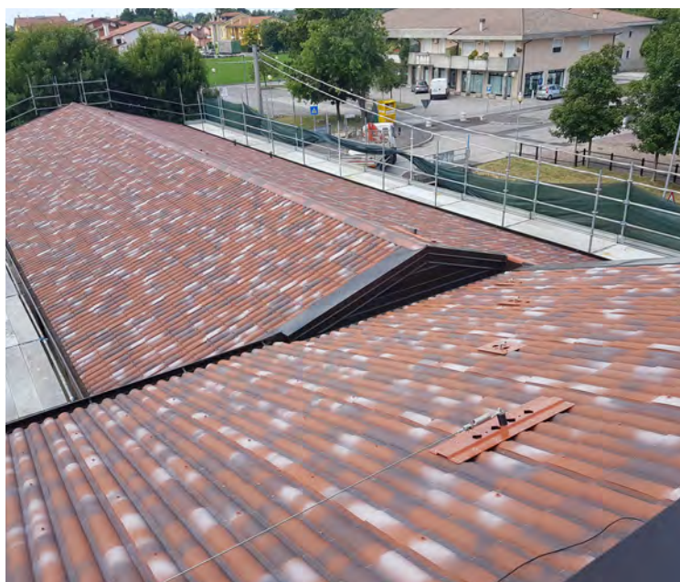
Pannelli sandwich Isometal (5G - in alto - SUPERCOPPO in basso) Isometal's sandwich panes (5G - above - SUPERCOPPO below)
